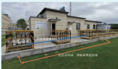
Reconstruction of open channel in Aohong Pharma
